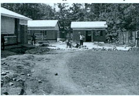
Parking area and distant kitchen
