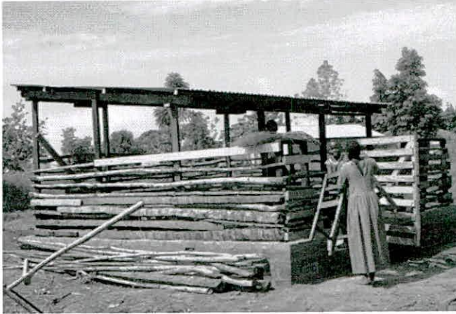
Pigpens were constructed in each of 7 parishes
