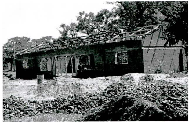
Wall and roof boards put in place
