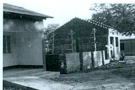
Restaurant structure in process
