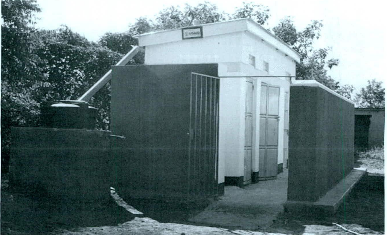
External view of the boys 'of a shower area and a latrine with 3 stances, one is fully wheelchair accessible
