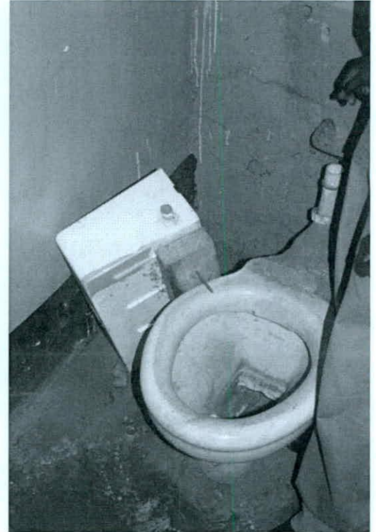
Toilet needing repair in CSLS office
