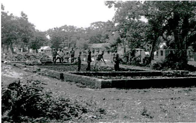
Working on the foundation of the building
