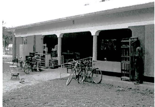
Completed building with on-going woodwork activity
